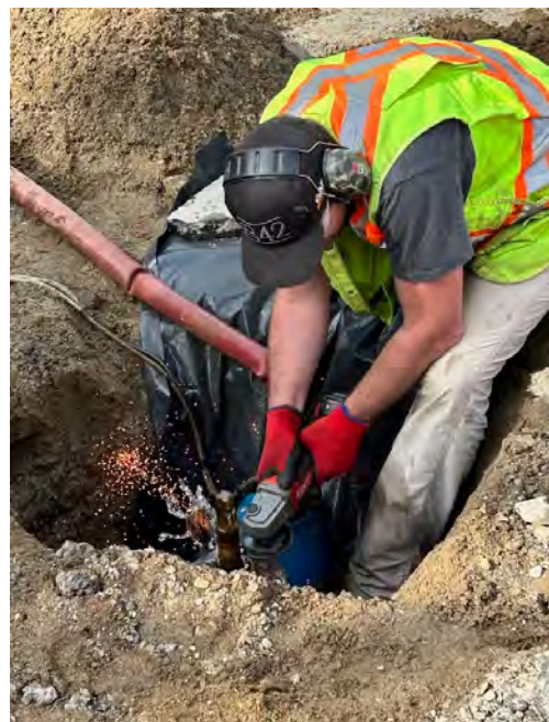
Leaking Water Valve Repair
