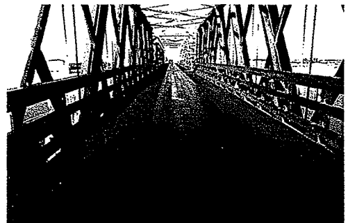
Westham Island Bridge.
